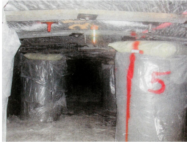
Figure 4 - Installation of pumpable cribs (Peng, 2007)
