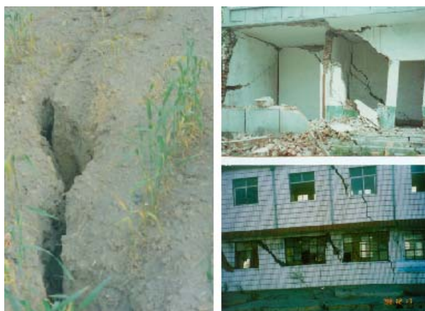
Figure 2 - Farmland and structures damaged by mining
